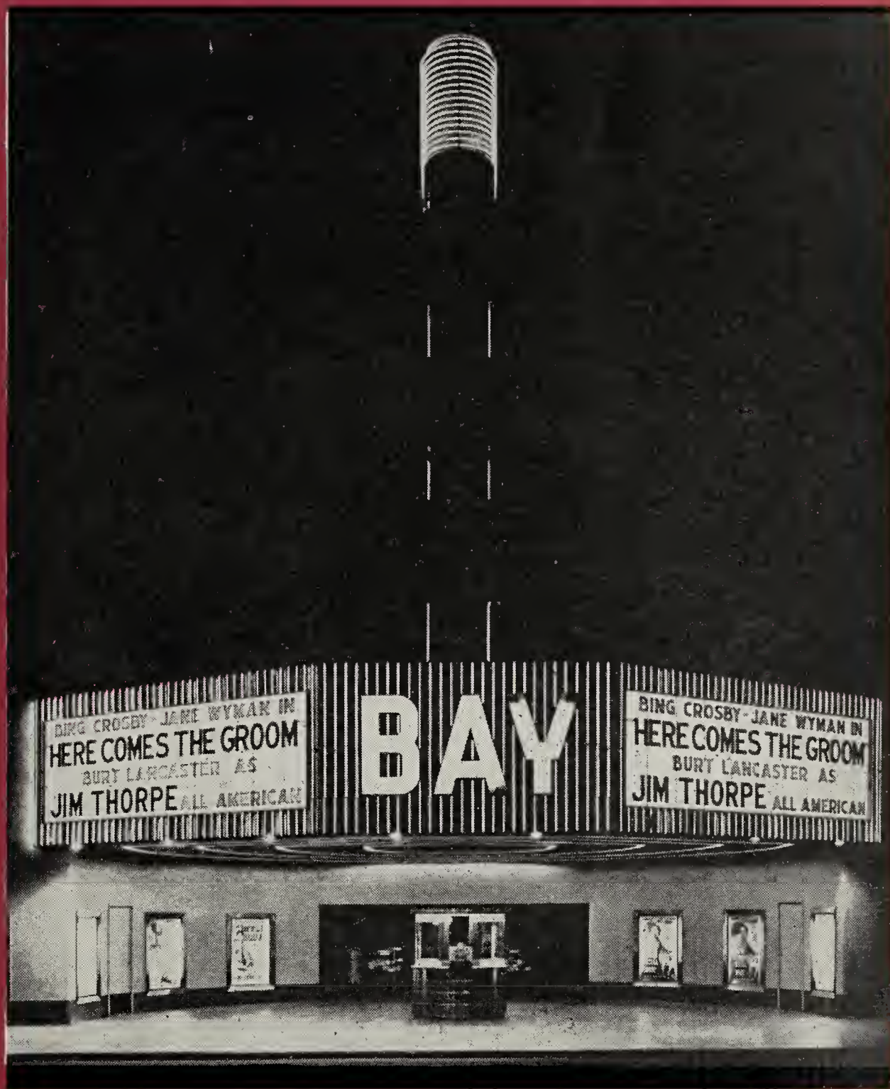
A most beautiful and effective front was accomplished by the Bay Theatre, National City, California, in the installation of attraction panels in a background of vertical neon tubing, which is particularly eye-catching at night. The Wagner attraction panels are each nineteen feet long.
